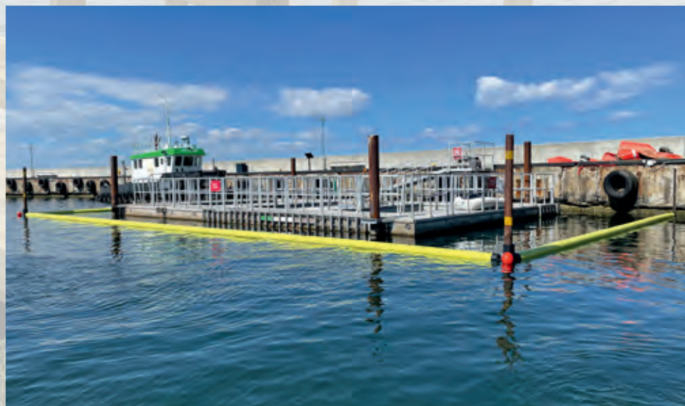
DTU Hundested Flydespærring platform
